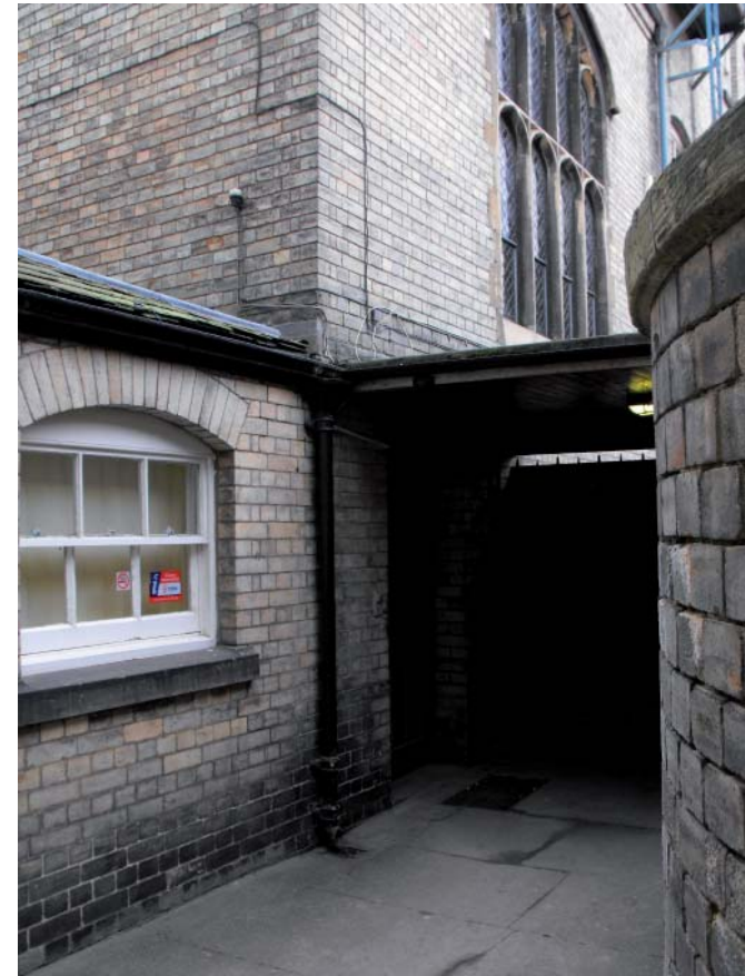
The existing Guildhall office entry is very unsatisfactory and not worthy of such an important Civic building. Accessibility is very poor.
