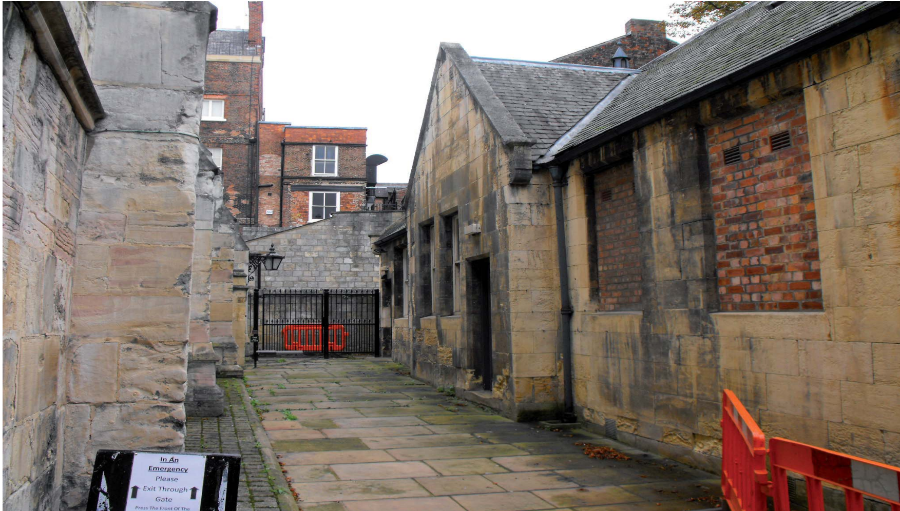
The East range and yard offer opportunity to form a glazed atrium space - providing separate access to toilets and meeting rooms from the Guildhall and Common Hall Yard.
