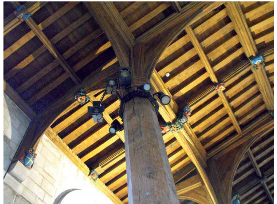
Interior timber frame structure of the Guild Hall
